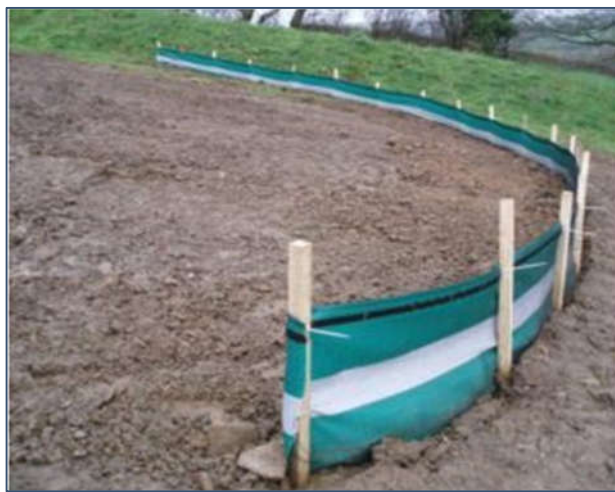
Plate 3-4 Embedded Silt Fence
