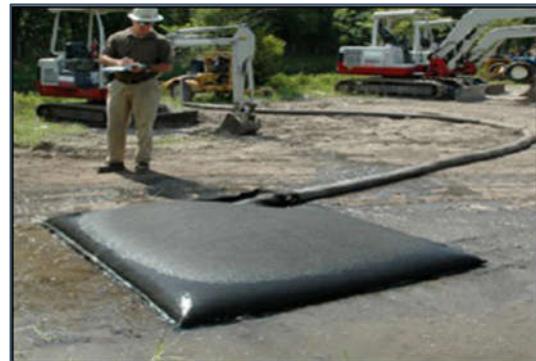
Plate 3-2 Silt Bag under inspection
