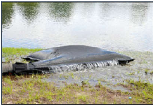
Plate 3-1 Silt Bag with water being pumped through.
